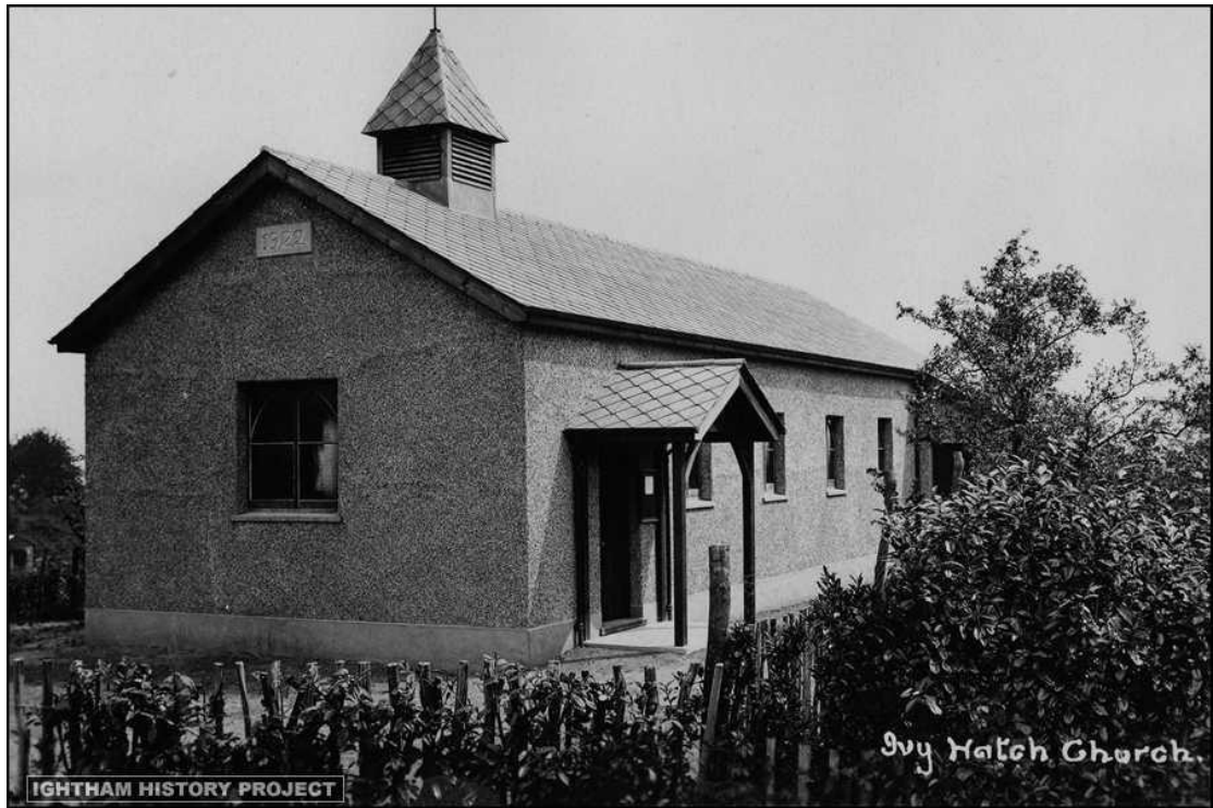
Fig. 1: Ivy Hatch Mission Church, Sevenoaks Source: Ightham History Project
